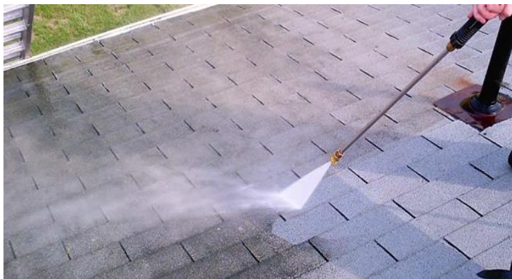
Power wash the roof and repiar all leak areas
