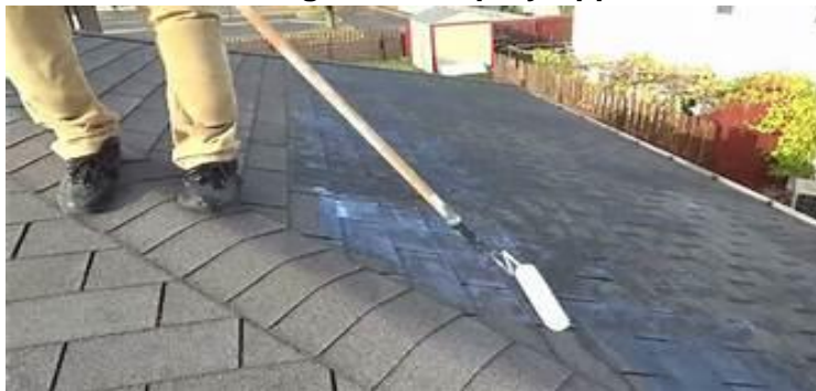
SG50 Shingle Saver Roller Applied
